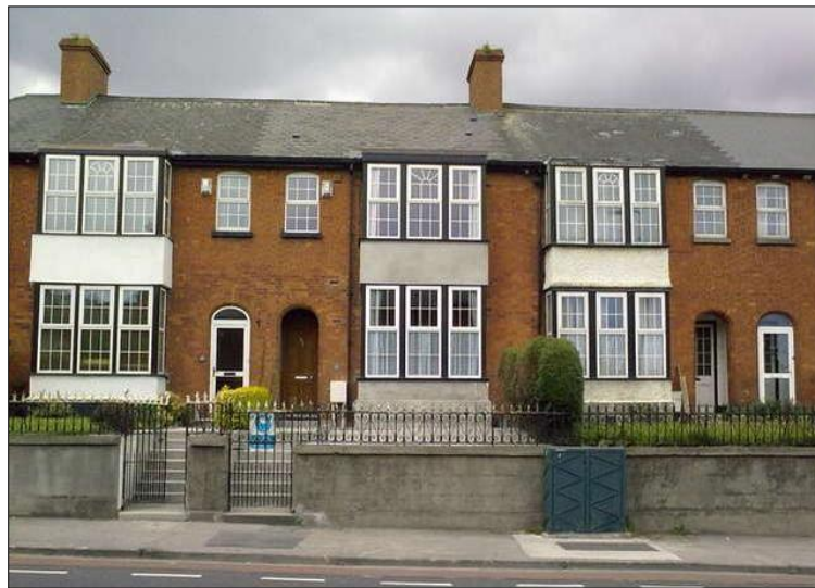
Figure 9.4 Properties on Botanic Road (Note steps to entrances)
